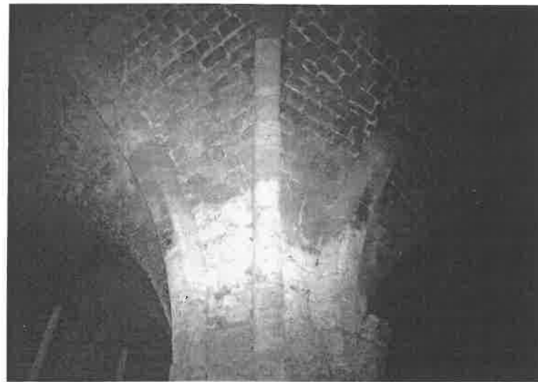
Fig. 5.5. Acre, Compound of the Knights of St. John, view of hall, showing springing of ribbed vaults, end of twelfth century. Photo: author.
