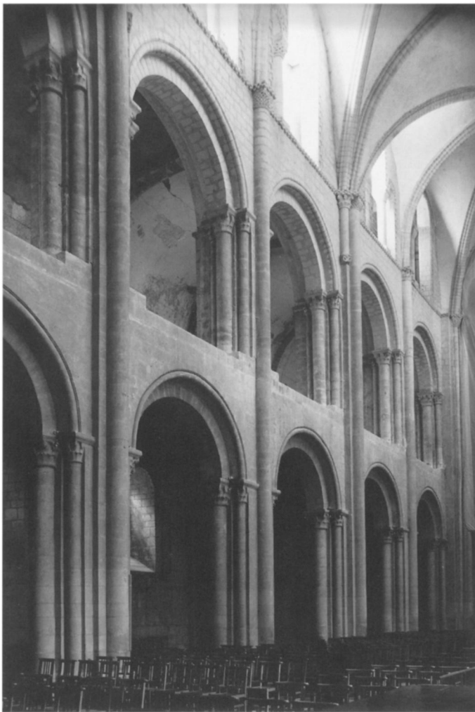
FIGURE 2. Caen, Saint-Étienne , nave elevation (photo: author).
