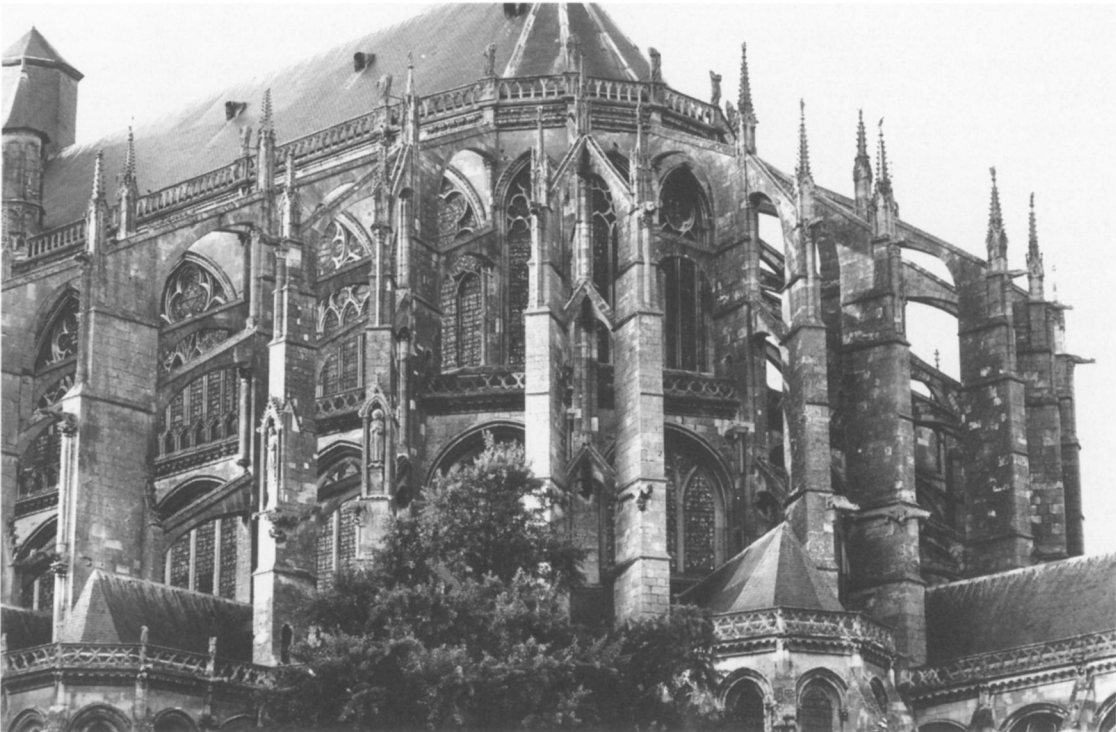
FIGURE 16. Le Mans, cathedral, choir buttresses (photo: author).
